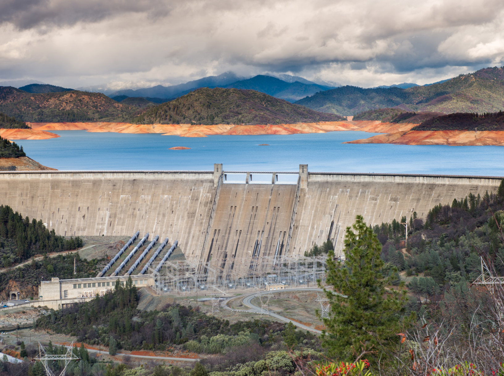
Shasta Dam, Calif. Courtesy Adobe Stock
